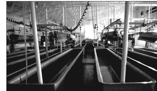
Start Tank Room
